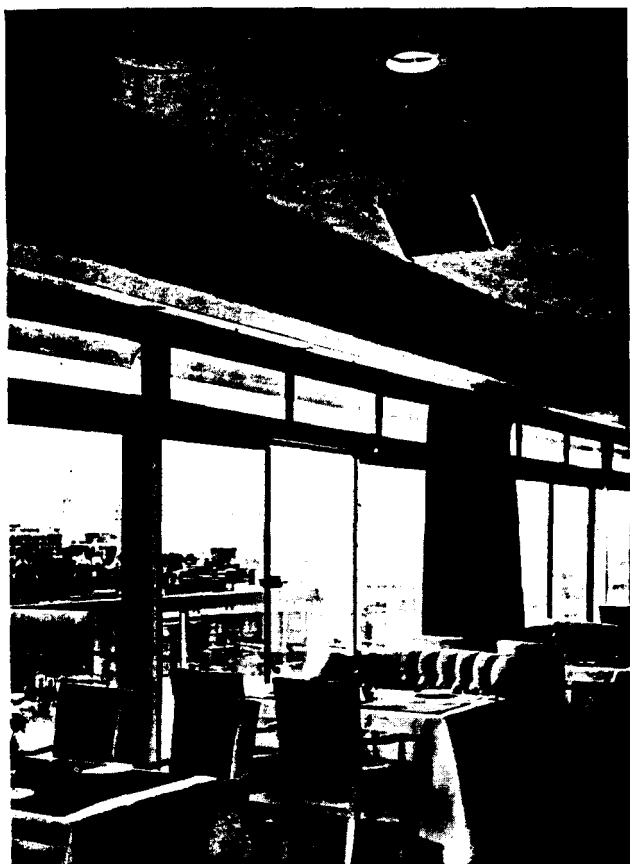
Fig. 1. Roof restaurant at Royal Garden Hotel, showing one of the bidirectional loudspeakers fixed to the ceiling in place of units behind the circular grilles in the ceiling.
